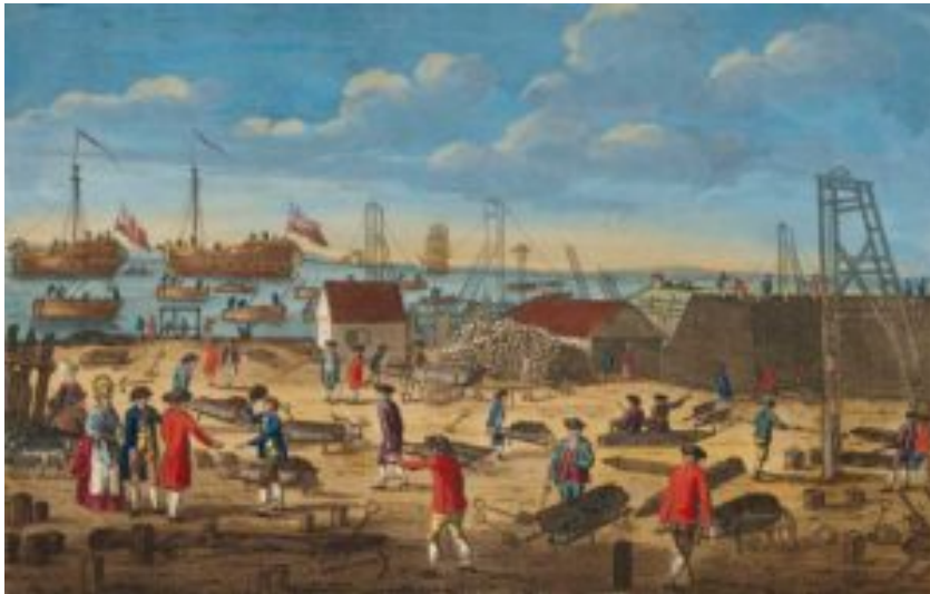
View near Woolwich in Kent showing convicts working in the shipyard, Museum of New South Wales.
